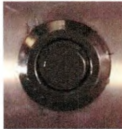
LDU Lock in Top Floor Door Jamb
