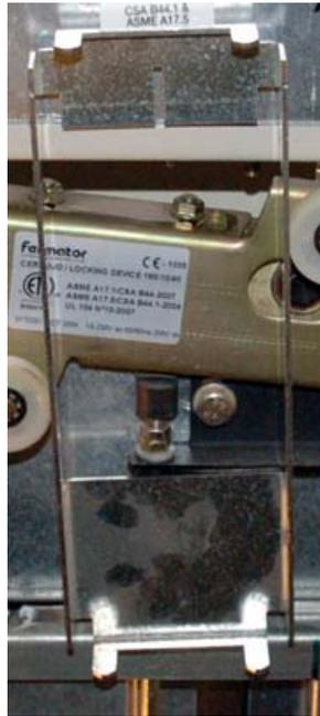
Alignment Tool Installed on Landing Door Interlock Release Rollers
