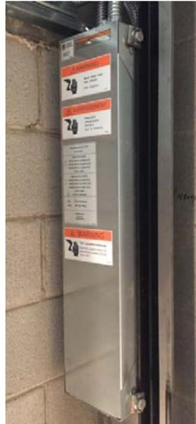
Transfer Switch Unit Mounted to Counterweight Guide Rail
